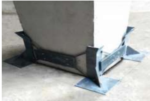
Fig. 2 Positioning of precast columns
