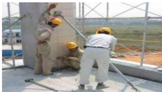
Fig. 3 Positioning and adjustment of vertical components
