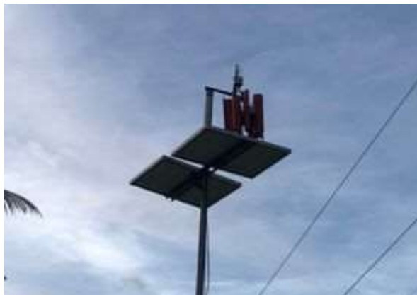
Figure 15. Solar Panels and Wind Turbine Installation
